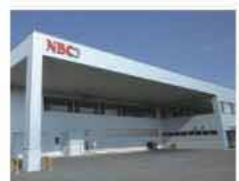
Shizuoka Kikugawa Factory
